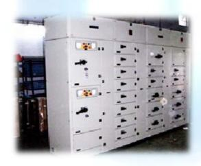
Power Distribution Equipments or Power Distribution Board is used for Electrical Power Distribution. In this ACB, MCCB, SDF, MCB etc are the main equipments. This receives supply from PCC. Power distribution board offers isolation and short circuit as basic protections. Other protections like over current, earth fault, earth leakage etc are offered on case to case basis.
